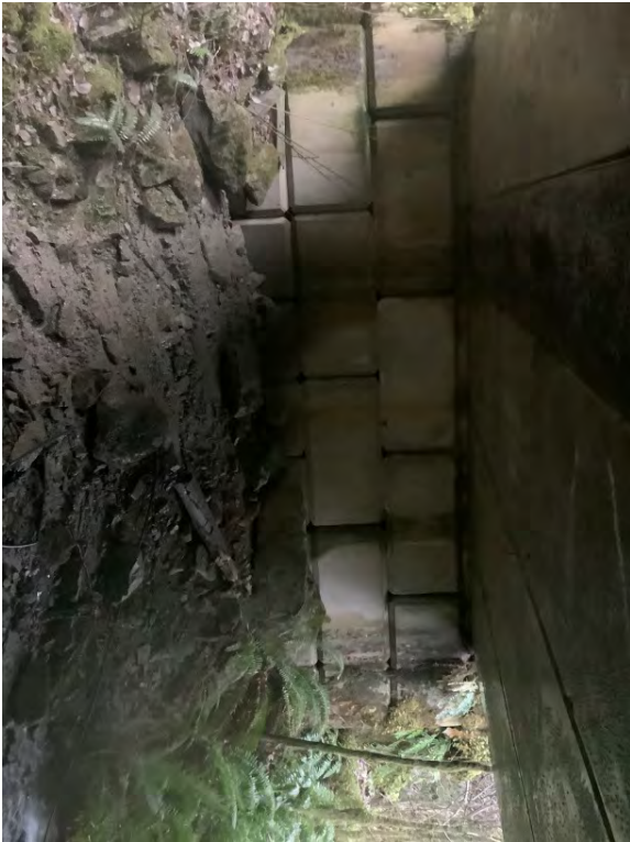
Left Bank Abutment when facing downstream
