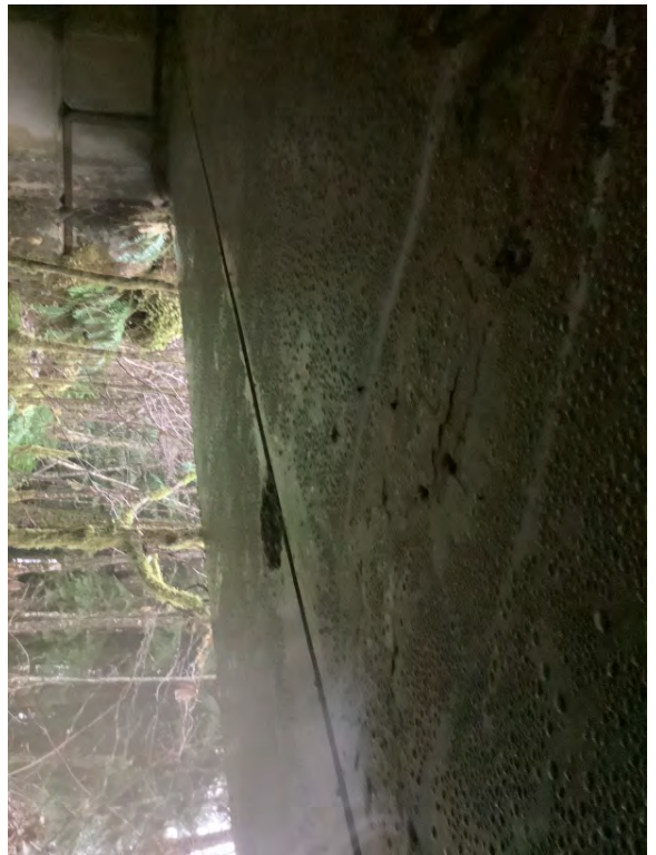
Superstructure-repaired area, minor chip DS right side
